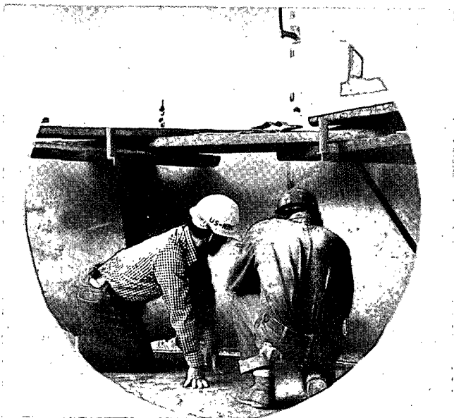
An NRC inspector examines welds on a reactor plant containment wall. Nearly one-third of the NRC's resources are committed to its inspection program and the task of verifying the safety of licensed nuclear activities. Most inspections are carried out by personnel assigned to NRC Regional Offices and on-site at nuclear facilities. (See Chapter 8.)
